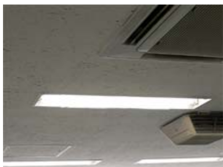
改善前 Before Improvement
